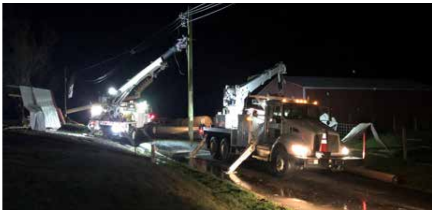
Nolin RECC crews repair a broken pole caused by wind damage from a March storm in Roanoke. Photo: Nolin RECC Line Technician Shaun Scherer
