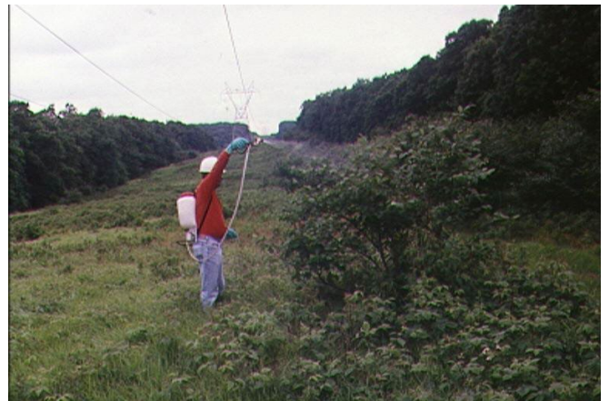
Selective Low Volume Foliar Using Backpack Sprayer
