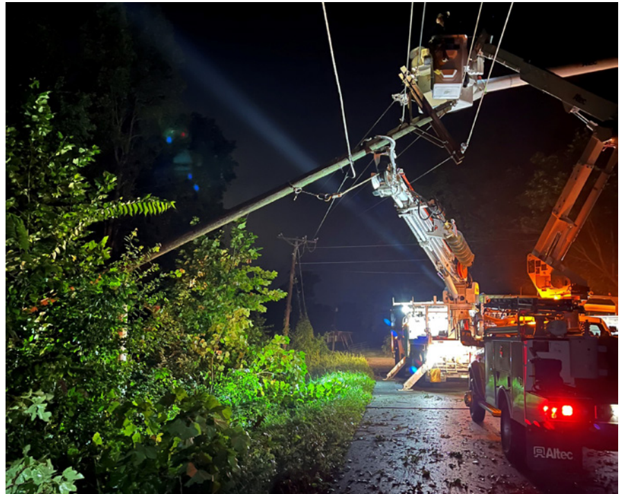
Nolin RECC lineworkers Preston Howell and Brandon Hurd work overnight to replace a pole broken by a late summer storm in Hardin County. Photo: Tyler Hornback
